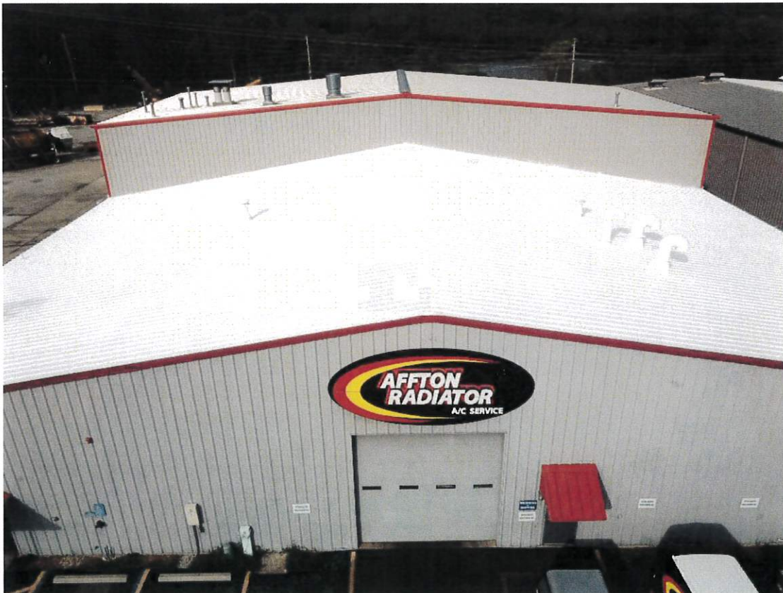
AFTER Roof is now 100% seamless and has a 20 year leak-free warranty.
