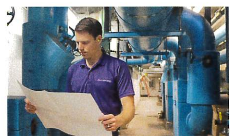
MECHANICAL, ELECTRICAL, PLUMBING
