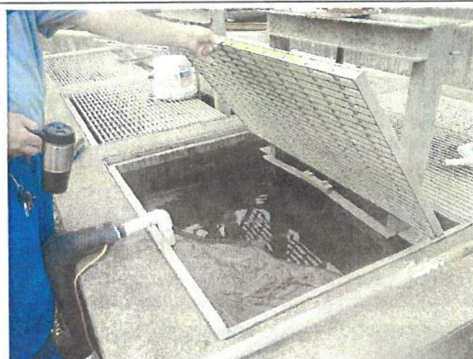
Photograph: #9 Taken By: Keith Forck Entity: Lake of the Ozarks WWTP #1 Permit: MO-0103241 Location: Lake of the Ozarks WWTP #1
