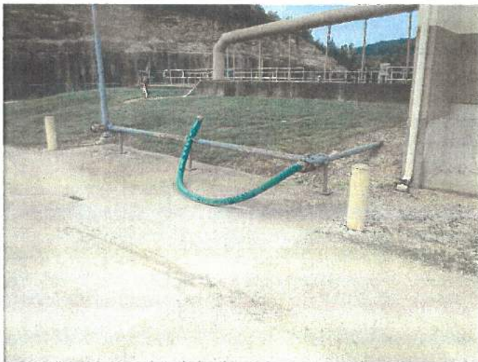
Photograph: #3 Taken By: Keith Forck Entity: Lake of the Ozarks WWTP #1 Permit: MO-0103241 Location: Lake of the Ozarks WWTP #1
