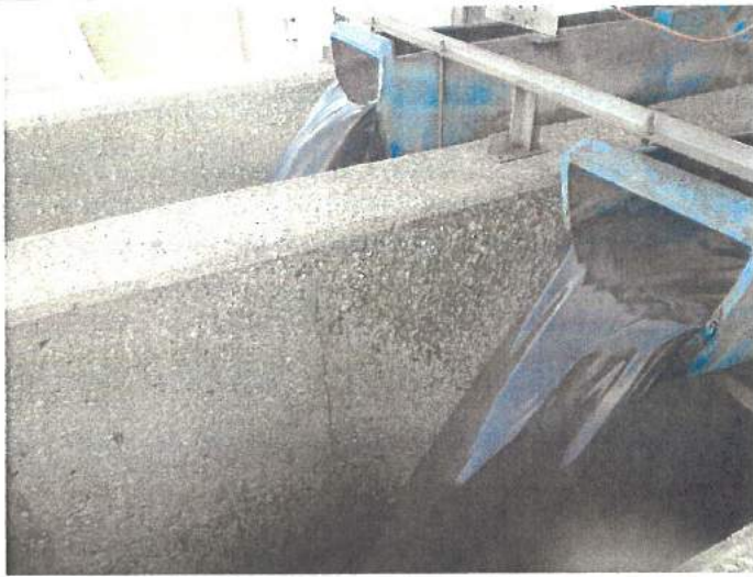
Photograph: #7 Taken By: Keith Forck Entity: Lake of the Ozarks WWTP #1 Permit: MO-0103241 Location: Lake of the Ozarks WWTP #1
