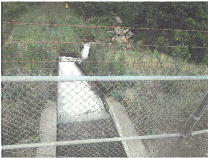
Photograph: #20 Taken By: Keith Forck Entity: Lake of the Ozarks WWTP #1 Permit: MO-0103241 Location: Lake of the Ozarks WWTP #1
