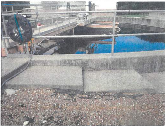
Photograph: #10 Taken By: Keith Forck Entity: Lake of the Ozarks WWTP #1 Permit: MO-0103241 Location: Lake of the Ozarks WWTP #1
