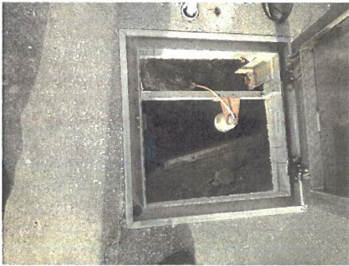
Photograph: #2 Taken By: Keith Forck Entity: Lake of the Ozarks WWTP #1 Permit: MO-0103241 Location: Lake of the Ozarks WWTP #1
