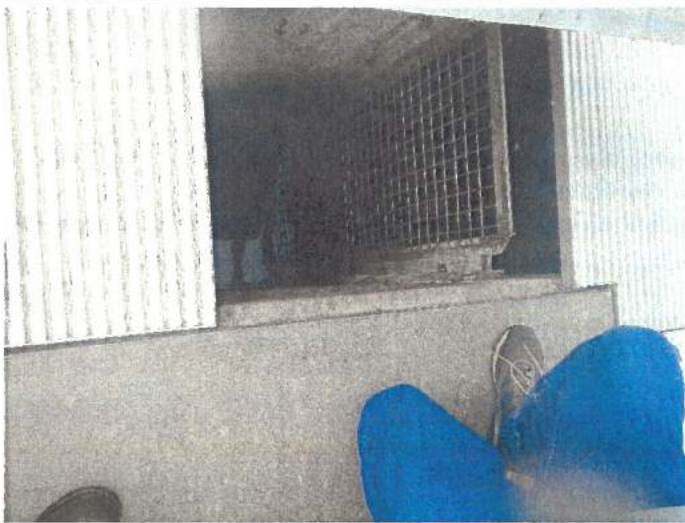
Photograph: #19 Taken By: Keith Forck Entity: Lake of the Ozarks WWTP #1 Permit: MO-0103241 Location: Lake of the Ozarks WWTP #1
