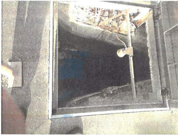
Photograph: #1 Taken By: Keith Forck Entity: Lake of the Ozarks WWTP #1 Permit: MO-0103241 Location: Lake of the Ozarks WWTP #1
