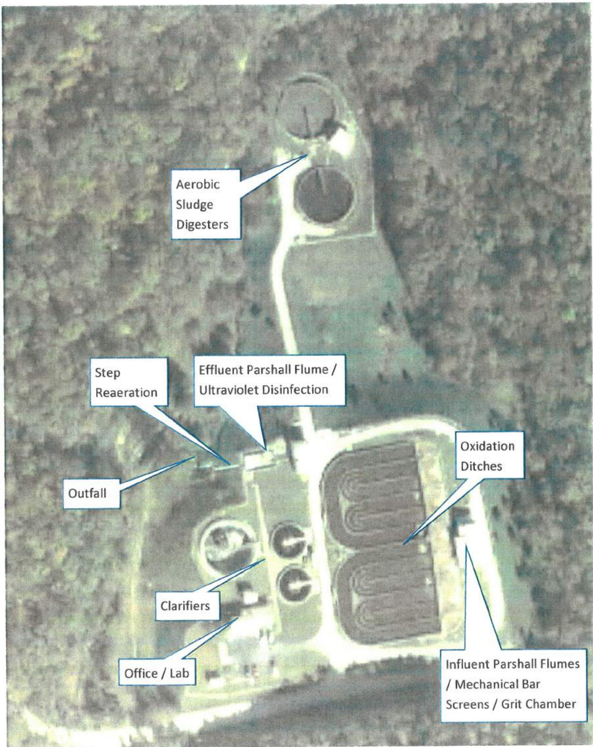
Figure 1: Aerial map of Lake of the Ozarks WWTP #1 courtesy of MapIT GIS System.
