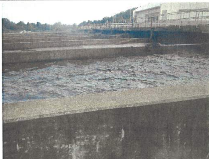
Photograph: #8 Taken By: Keith Forck Entity: Lake of the Ozarks WWTP #1 Permit: MO-0103241 Location: Lake of the Ozarks WWTP #1
