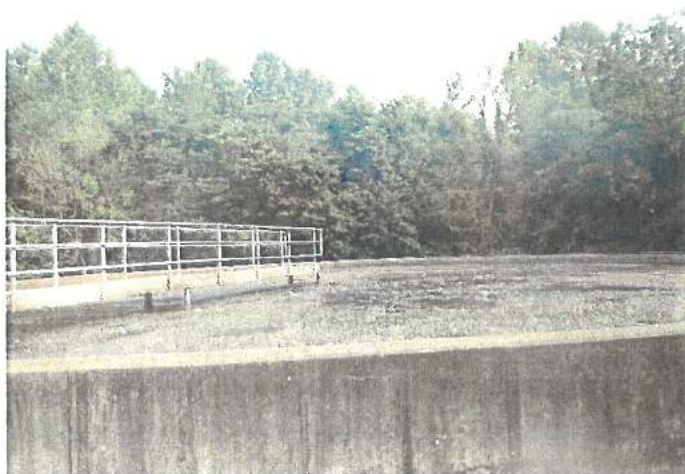
Photograph: #21 Taken By: Keith Forck Entity: Lake of the Ozarks WWTP #1 Permit: MO-0103241 Location: Lake of the Ozarks WWTP #1
