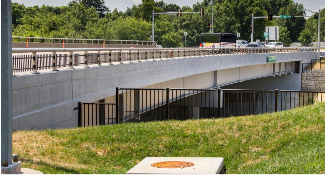
FIG. 3.1.2: CHESTERFIELD PARKWAY BRIDGE AFTER COATING BEAMS AND STAINING CONCRETE
