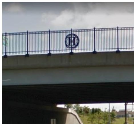
FIG 3.4.3: CUSTOMIZED CITY LOGO IN PEDESTRIAN RAILING ON BRIDGE
