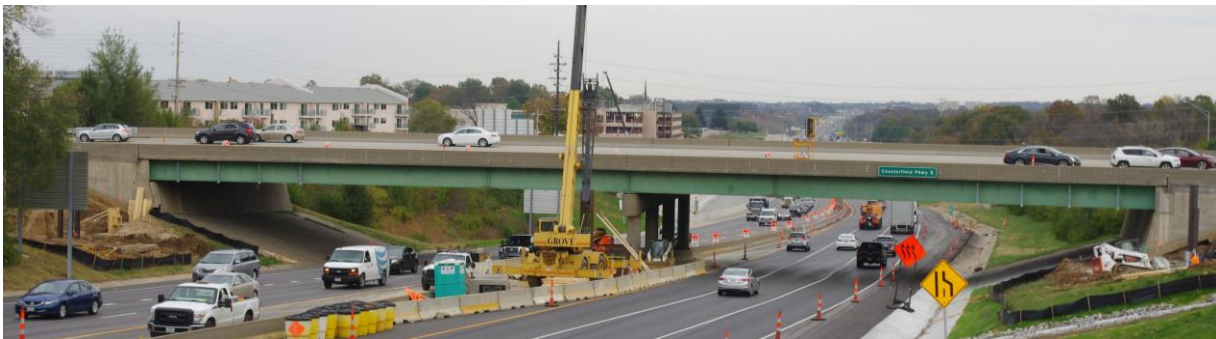
FIG. 3.1.1: CHESTERFIELD PARKWAY BRIDGE (PRE-IMPROVEMENTS)
