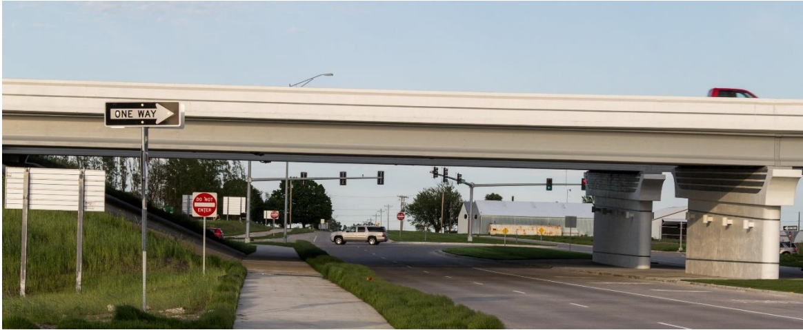
FIG. 3.1.4: I-35 BRIDGE UTILIZING TWO COLORS OF CONCRETE STAIN
