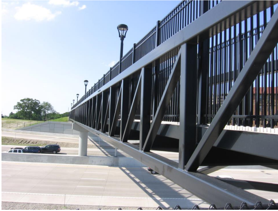
FIG. 2.4.1: STEEL TRUSS PEDESTRIAN BRIDGE
