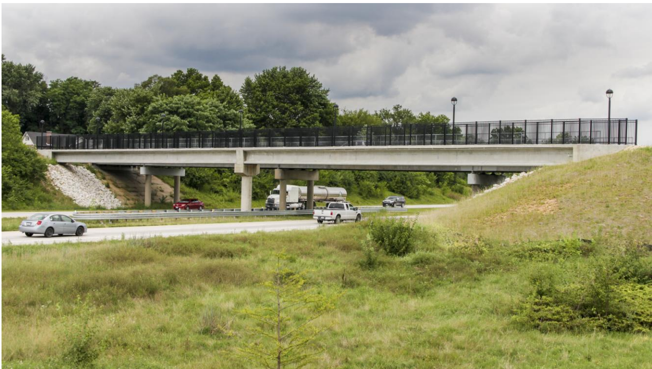
FIG. 2.4.2: PRESTRESSED I-GIRDER PEDESTRIAN BRIDGE
